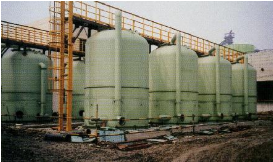
Photo of fiber filters installation site
